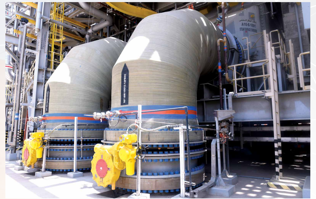
Nonmetallic piping at Jazan Refinery Complex.
